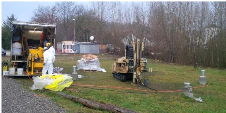
Figure 1. Direct injection application of EHC<sup>®</sup> Reagent
